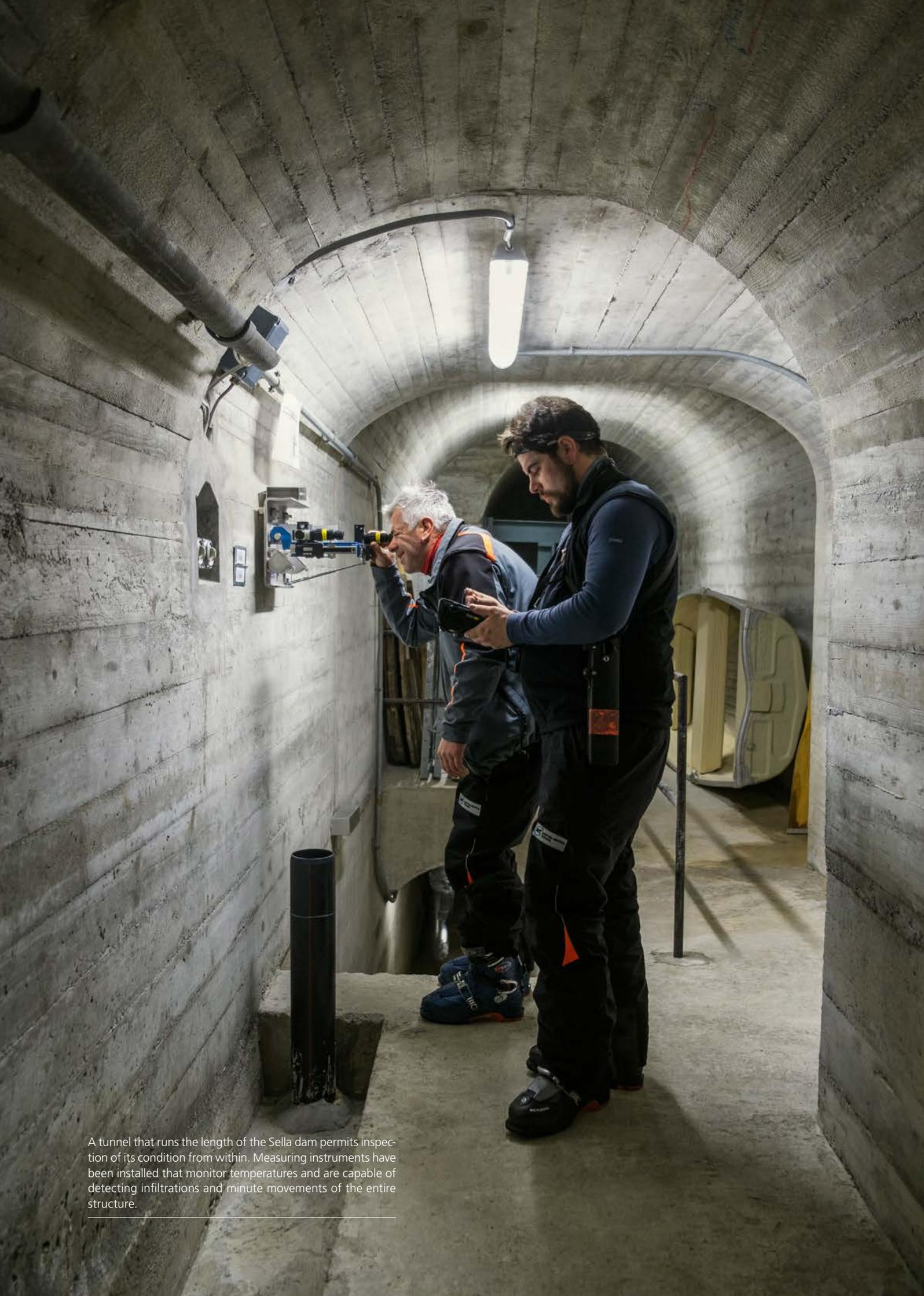
A tunnel that runs the length of the Sella dam permits inspection of its condition from within. Measuring instruments have been installed that monitor temperatures and are capable of detecting infiltrations and minute movements of the entire structure.
