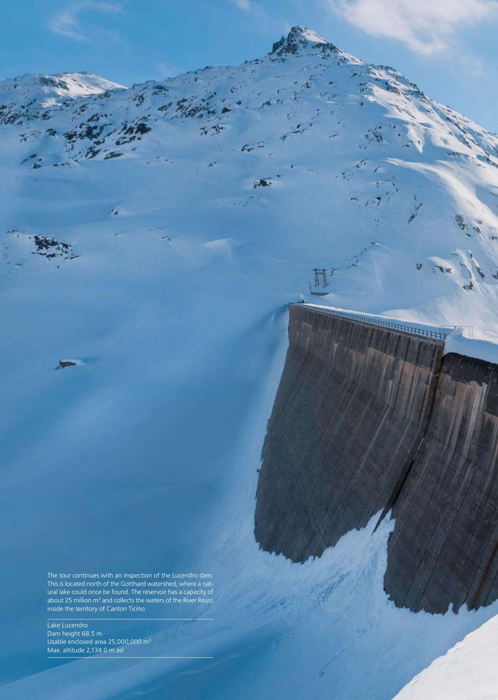
The tour continues with an inspection of the Lucendro dam. This is located north of the Gotthard watershed, where a natural lake could once be found. The reservoir has a capacity of about 25 million m<sup>3</sup> and collects the waters of the River Reuss inside the territory of Canton Ticino.
