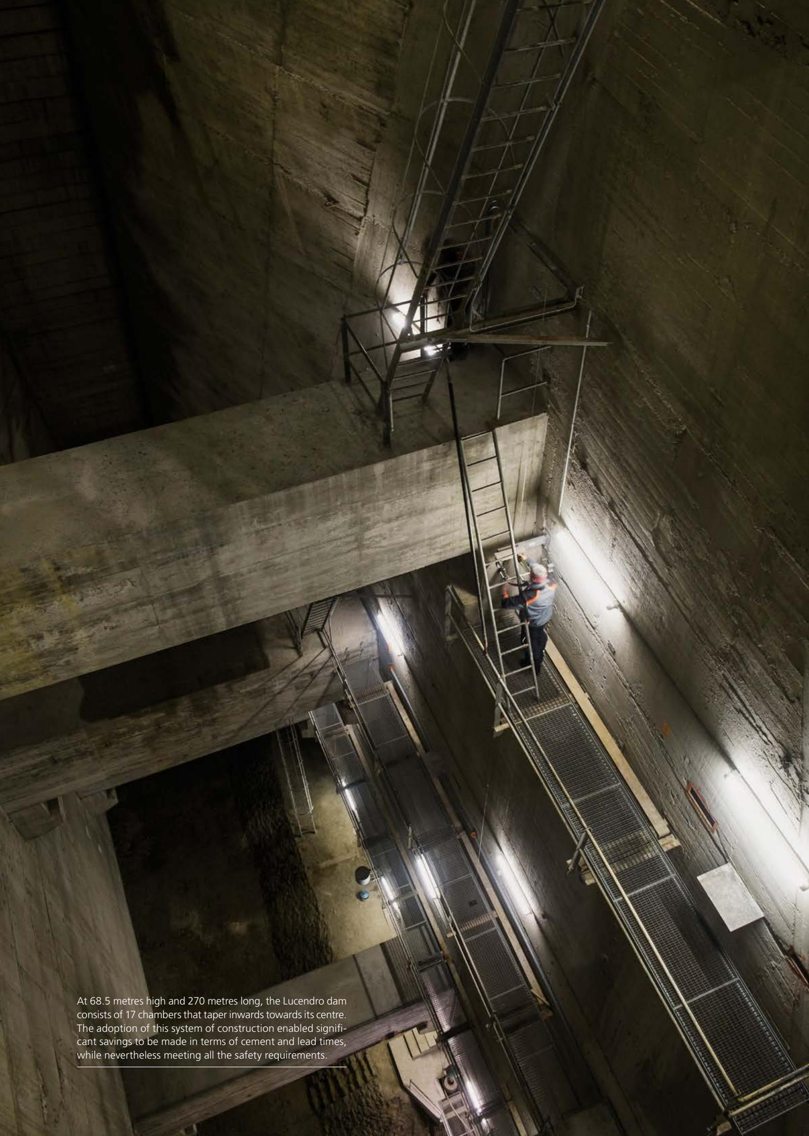
At 68.5 metres high and 270 metres long, the Lucendro dam consists of 17 chambers that taper inwards towards its centre. The adoption of this system of construction enabled significant savings to be made in terms of cement and lead times, while nevertheless meeting all the safety requirements.
