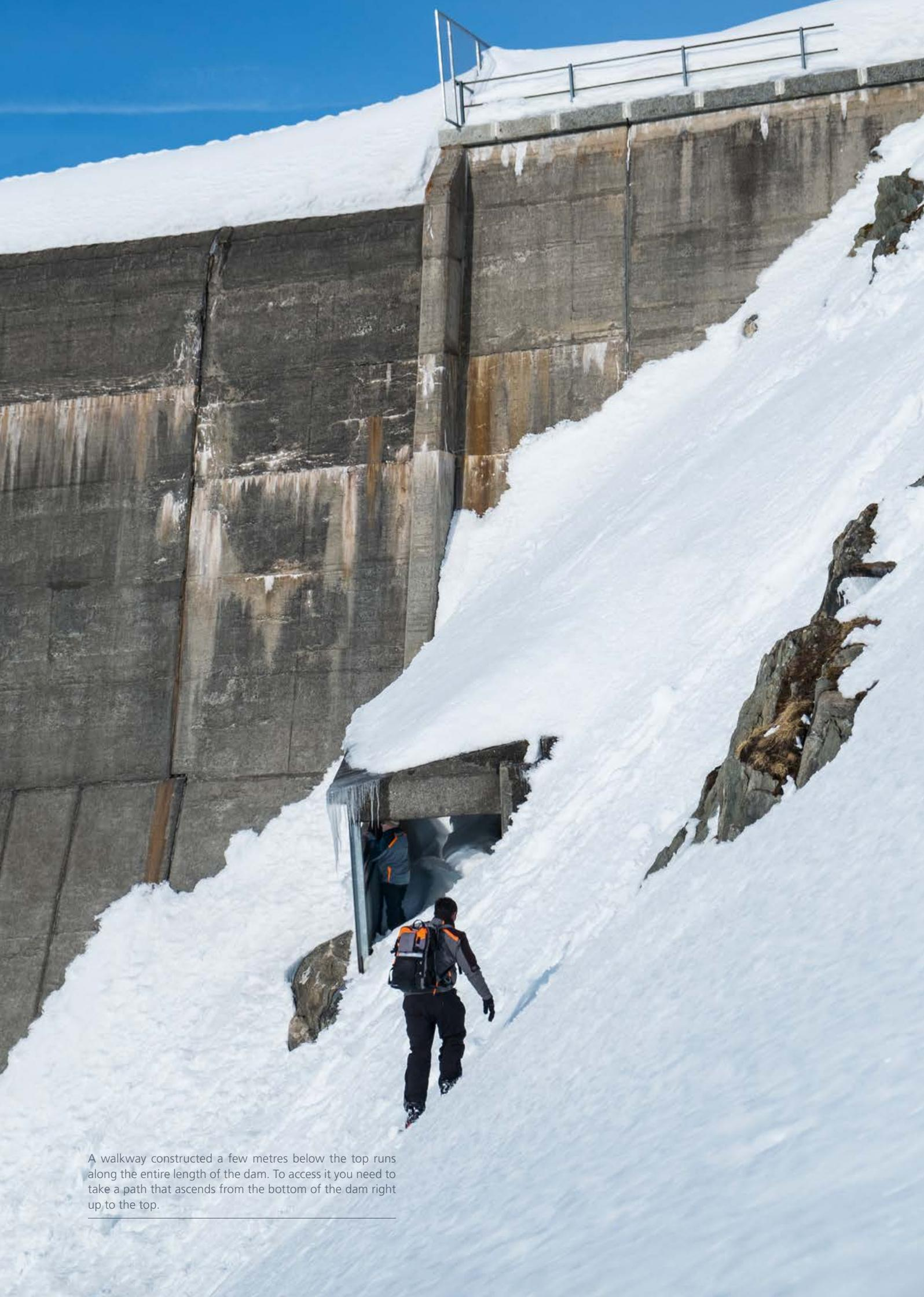
A walkway constructed a few metres below the top runs along the entire length of the dam. To access it you need to take a path that ascends from the bottom of the dam right up to the top.
