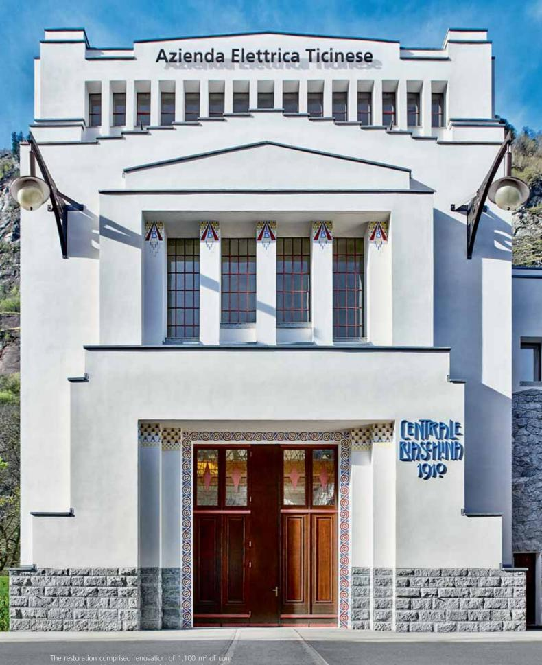
The restoration comprised renovation of 1,100 m<sup>2</sup> of concrete render, washing and cleaning of the stonework, repainting of the external wood and ironwork, and repair of the original decorative features.
